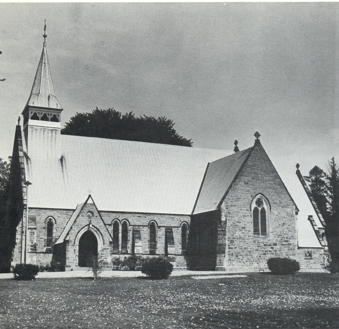
St. Luke's Church, Beacon. Designers Vaux and Withers were careful to place the main door in the "correct English" location on the south side, and the arboreal-minded Sargent family completed the perfect mid-Victorian setting by planting specimen shade trees in the churchyard.
