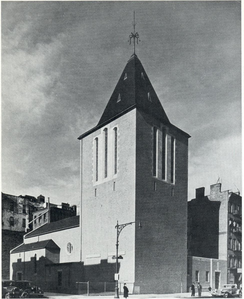
Manhattan's Church of the Epiphany, located on York Avenue where Bishop Manning said it should be. Architects: Wyeth and King.
