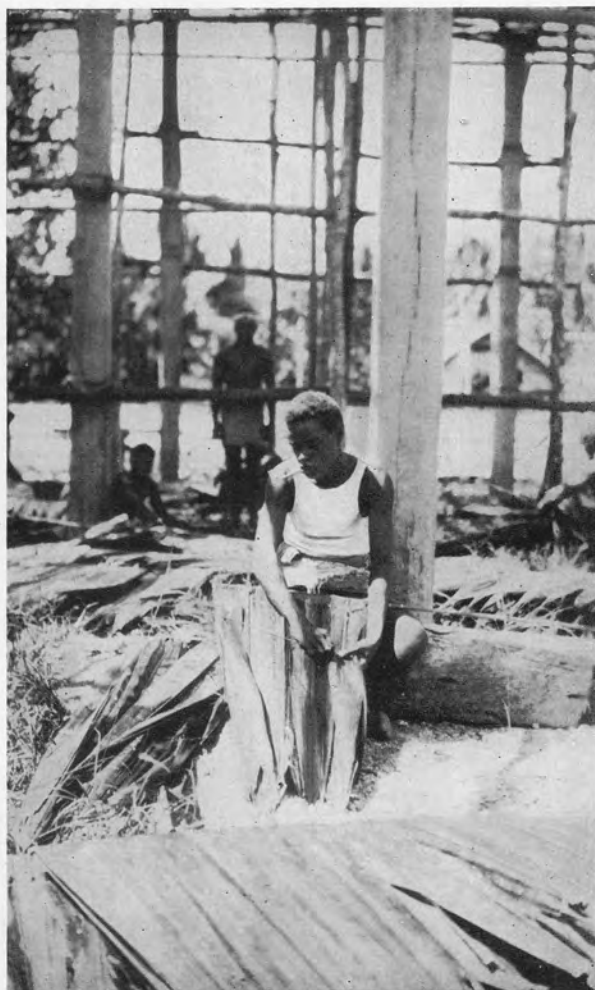
MAKING THATCH FOR THE CATHEDRAL ROOF.
